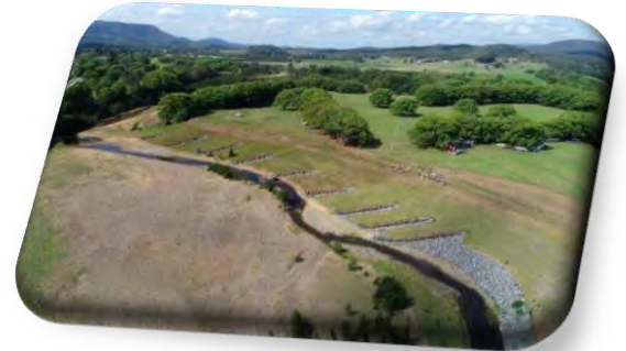
above: pile forest Mary River
